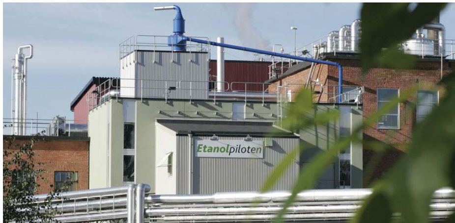
SEKAB cellulose ethanol R&D Pilot Plant
